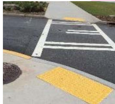
Wheelchair accessible ramp
