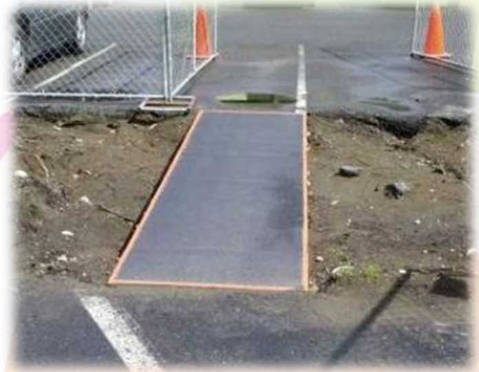
Ramp with slip resistant coating
